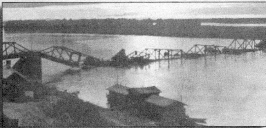
The Germans destroyed this bridge over the Erif River prior to the Division's arrival at the Rhine. Photo: Paul Priest
